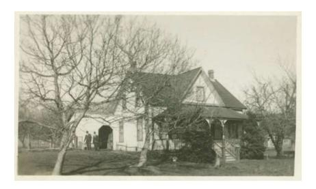
"1930's form": modifications made between 1920 and 1970 which included enclosing and extension of the south porch, expansion of the main floor, shed extensions to the north and south sides of the roof, and addition of a carport on the north.
