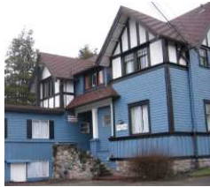
The Green-Armytage House before restoration
