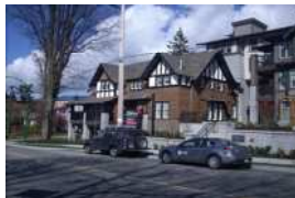
The house after restoration
